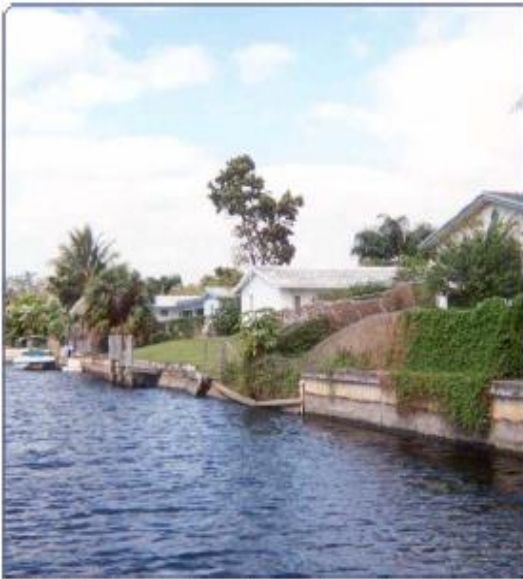
Failed bulkhead due to inadequate embedment of wall.
