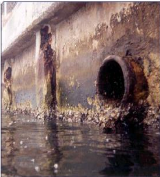
Deteriorated concrete pile/panel bulkhead. Note storm sewer outfall through bulkhead.
